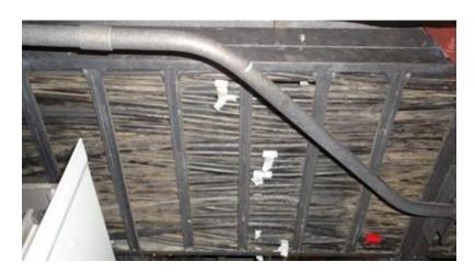
Harvesting field aged cables for additional temperature and radiation testing
