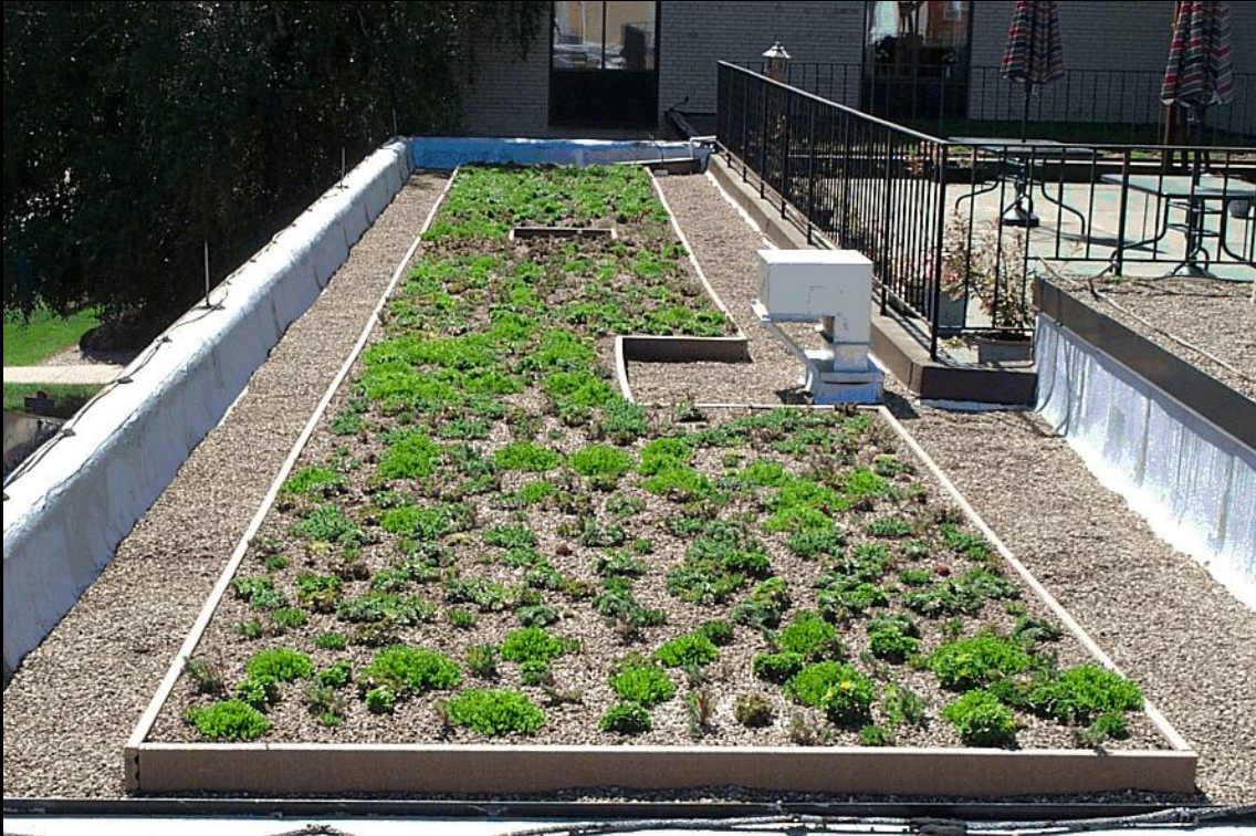
Green roof at nursing home
