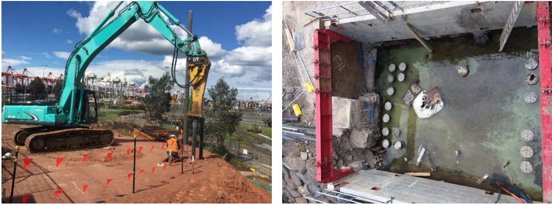
Figure 2 – Piling Rig (East Abutment) & Installed Group (East Pier)
