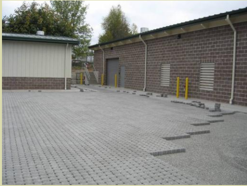
Wastewater Treatment Plant, Winlock, WA
