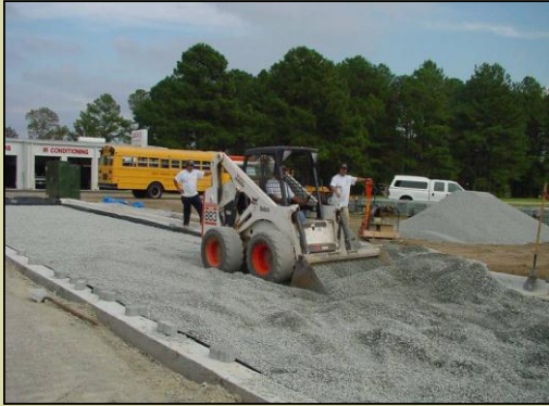
Final grading of base material
