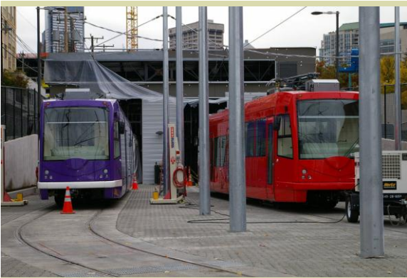
South Lake Union Street Car Facility
