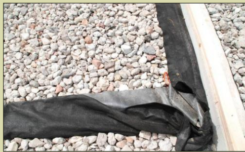
Impermeable EPDM (or equivalent) liner
