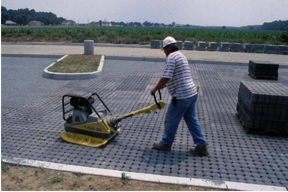
Compact before sweeping in aggregate
