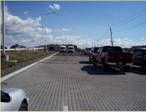
Tacoma Landfill Pervious Pave Demo
