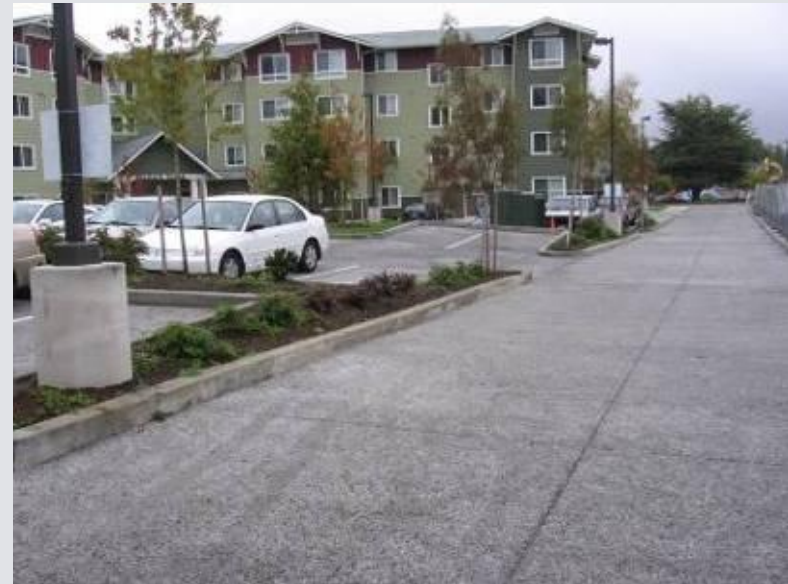
Pervious Concrete Parking Lot, Seattle
