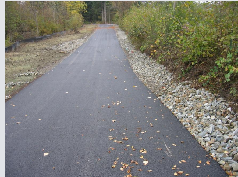
Porous Asphalt Drive, Pierce County
