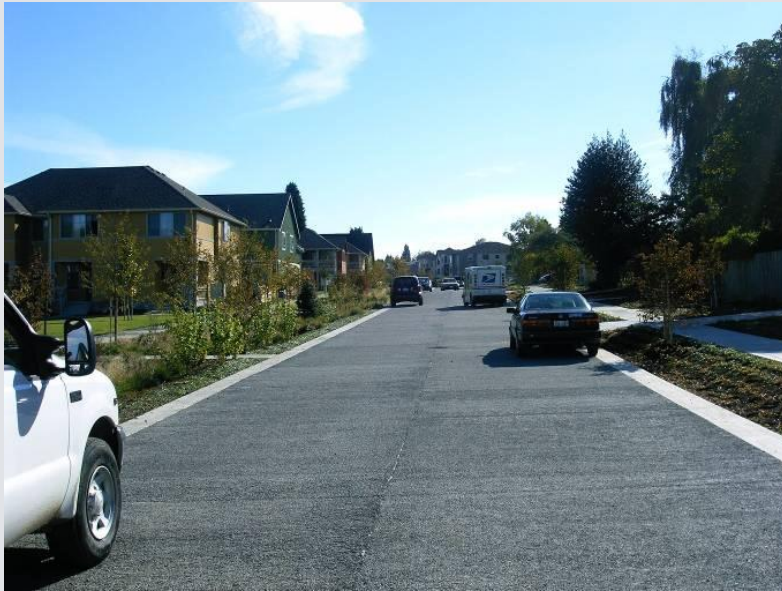
32 nd Ave. SW, Seattle. Pervious Concrete (2005 – 8" PPCC over 18" subbase)
