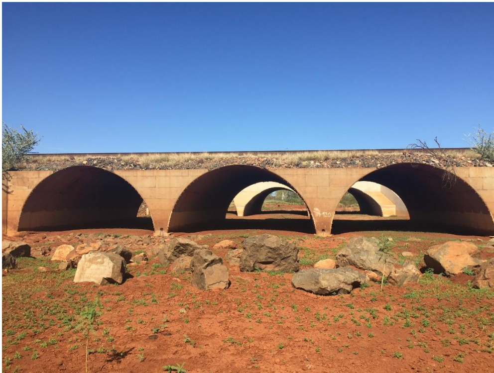
Figure 2 Original Bridge before relining
