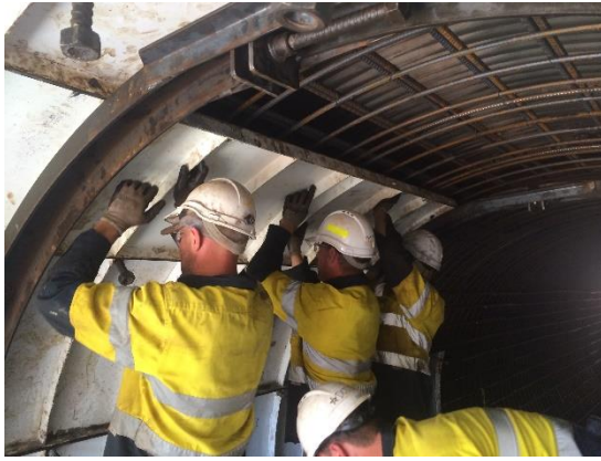
Figure 11 Installing Formwork Panels
