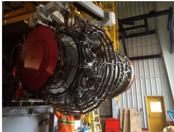
Figure 20: Parkway “C” RB21124GT-DLE Engine being hoisted into enclosure
