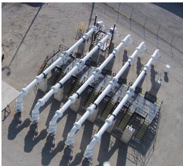
Figure 15: Aerial View of Completed Meter Runs
