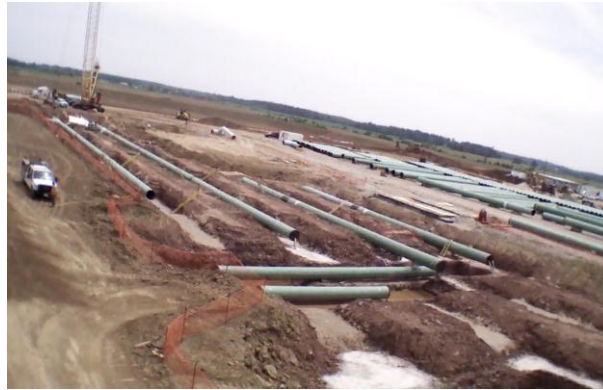
Figure 14: Aerial View of Station Headers in Early Phases of Construction
