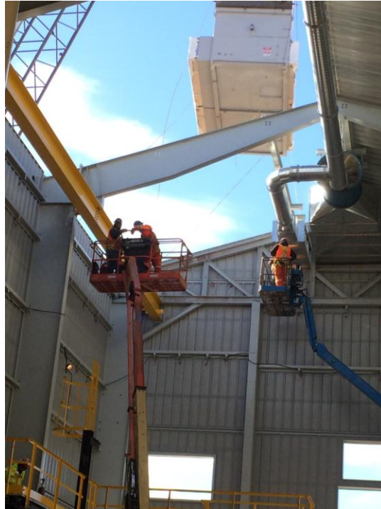
Figure 19: Installation of Parkway “D” Lube Oil Cooler through building roof
