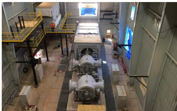
Figure 7: Parkway “D” Compressor Installed
