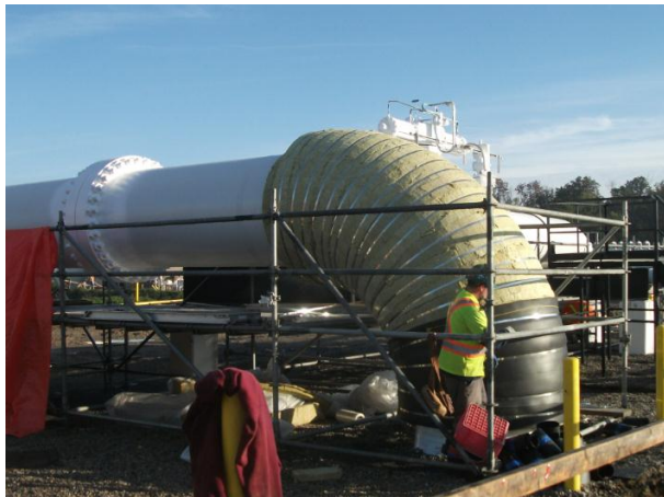
Figure 11: Acoustic Insulation Installation
