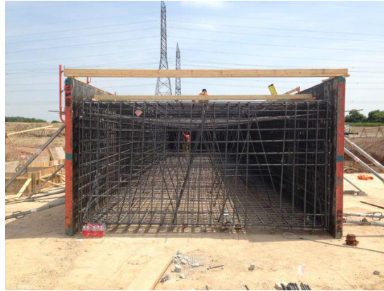
Figure 16: Parkway “D” compressor block rebar cages, June 2014
