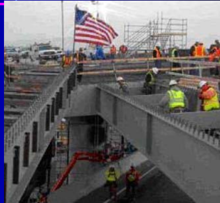
Last girder installed at the jobsite
