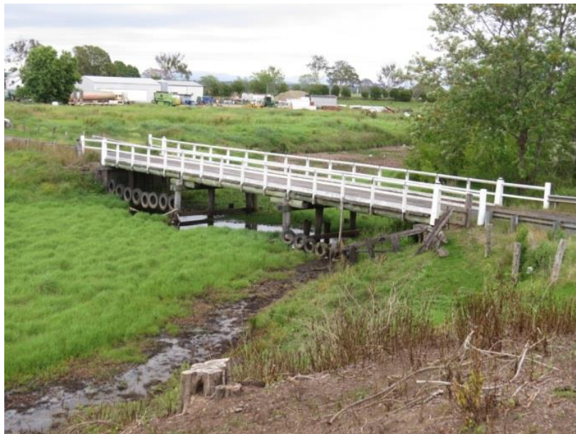
Typical three span timber beam bridge, Butterfactory Lane, Grafton
