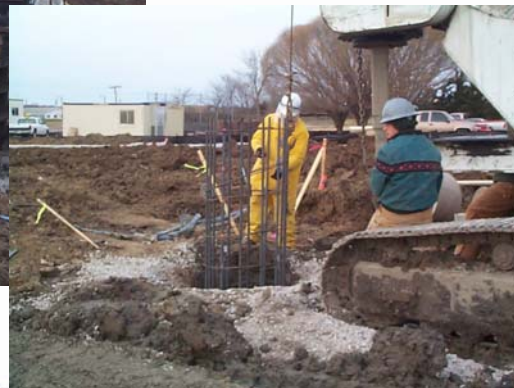
Setting rebar for concrete piers
