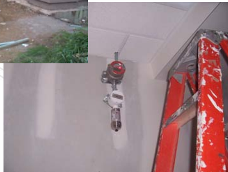
Interior-Mounted Ultima X Gas Methane Monitor & Alarm
