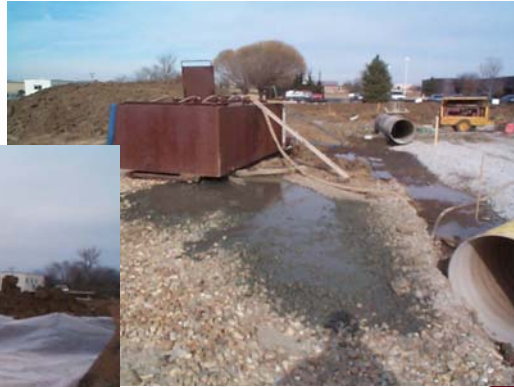
Groundwater Waste (Pumped from piers)
