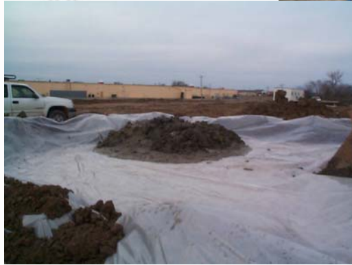
Solid Waste (Drill cuttings for piers)
