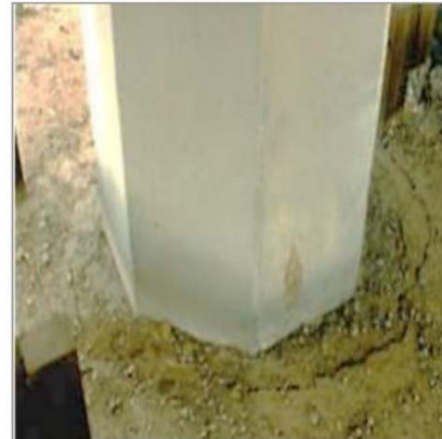
Figure 100: Ground movement indicating possible foundation problems ( INDOT ) ACTION: Report findings immediately and request Stage 2 Inspection.
