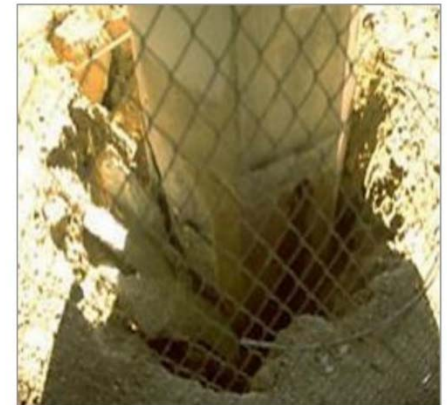
Figure 100: Ground movement indicating possible foundation problems ( INDOT ) ACTION: Report findings immediately and request Stage 2 Inspection.
