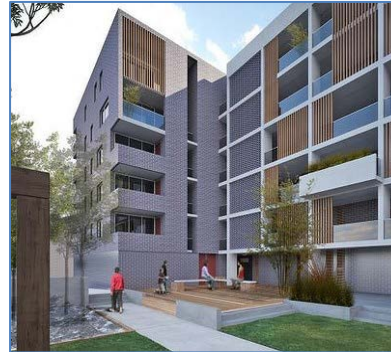
CityWest Housing – North Eveleigh project, Sydney – completed 2015
