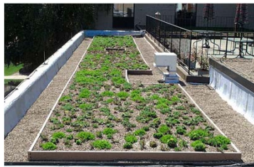
Green roof at nursing home
