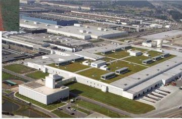
Ford Rouge River Plant Source: www.greenroofs.com
