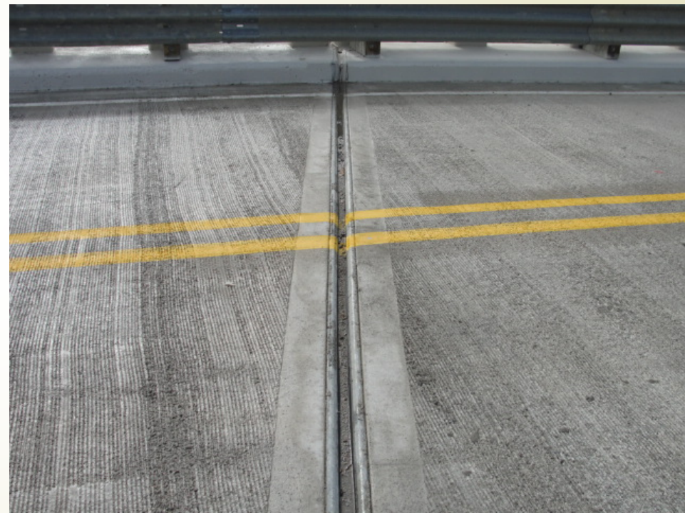
New Expansion Joints
