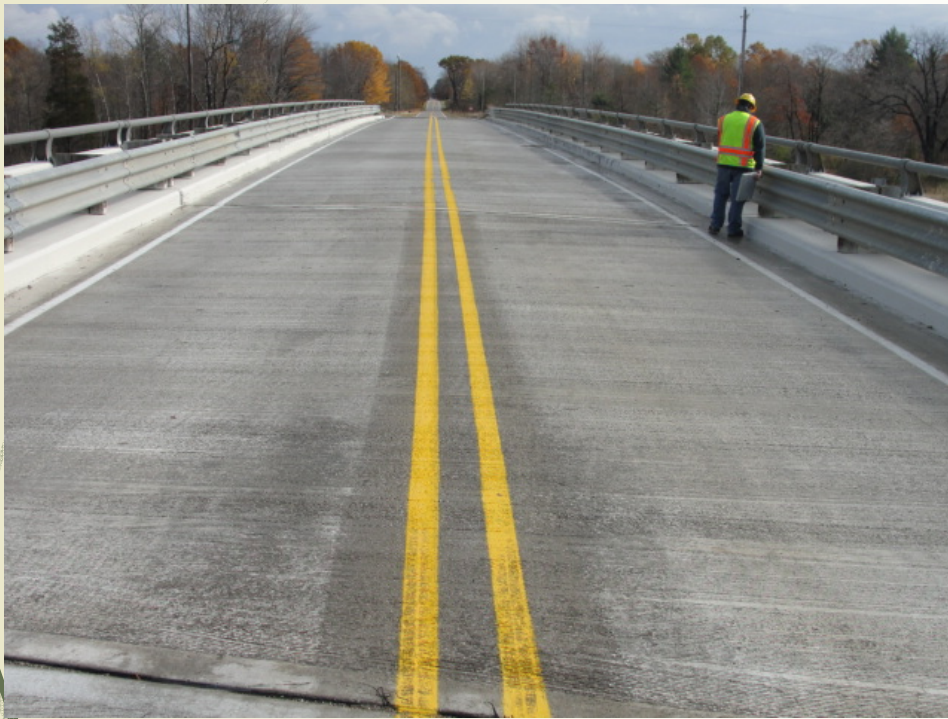
New concrete deck surface
