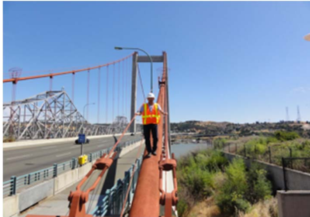
Maintenance Cables (New Carquinez)
