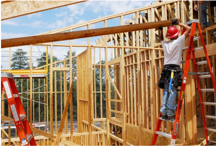
Conventional building construction
