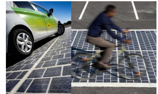
French Colas/INES solar highways wirelessly charging electric cars
