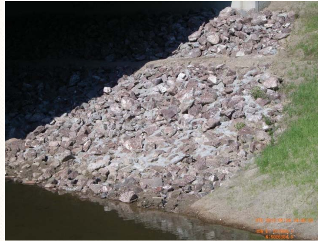
(Matrix Riprap, partially grouted riprap)
