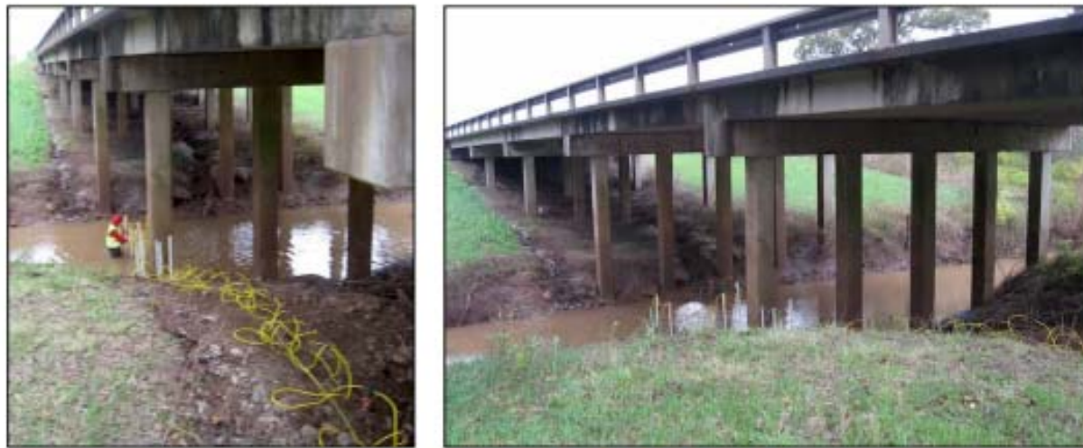
Figure 11-6. Bridge 14 ERI Fieldwork.
