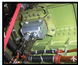
Aft Compartment Hydrogen Monitoring
