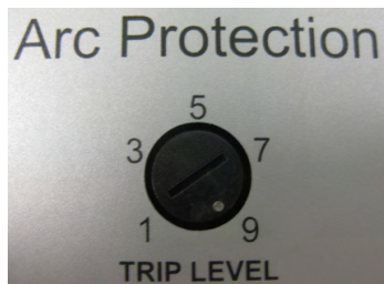
Fig. 6. Arc protection analog setting knob
