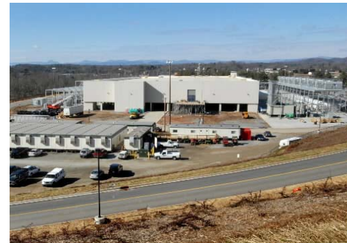
Google Data Center in Lenoir, NC circa 2005
