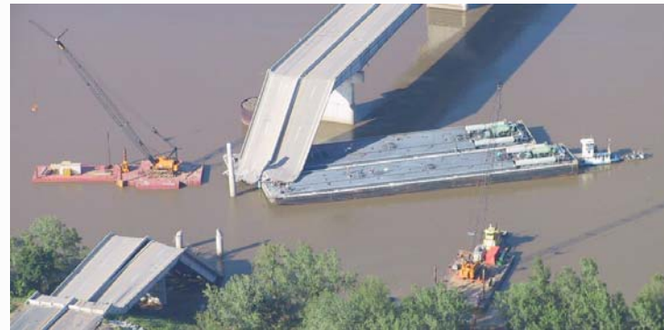
Structural failure of bridge resulting from Structural Defects
