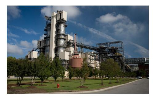
The largest paper machine converted to a fluff pulp dryer in 2010. Mill currently 1,250 admt per day <u>softwood</u> fluff pulp from the two fiberlines.
