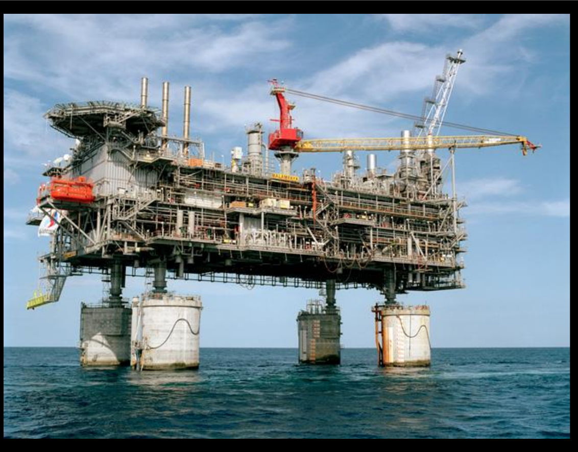
Malampaya Natural Gas Platform
