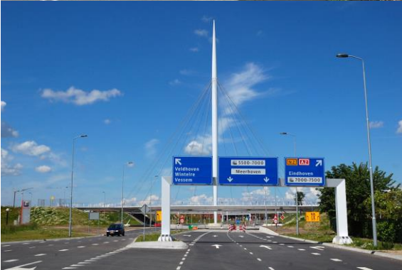
Fig. 12. Design for 250 kN collision force collision portals
