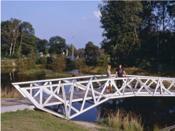
Fig. 3. Footbridge referring to local railway history excavated existing dam
