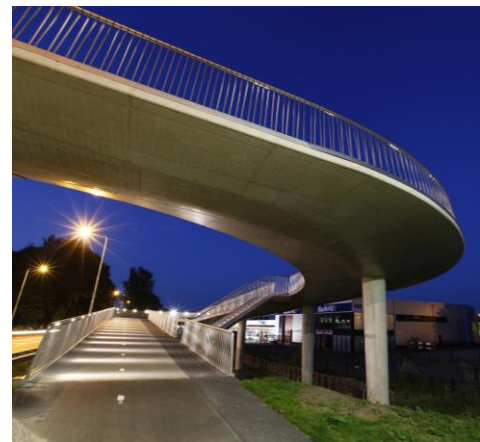
Fig.11. Ramp in complex
