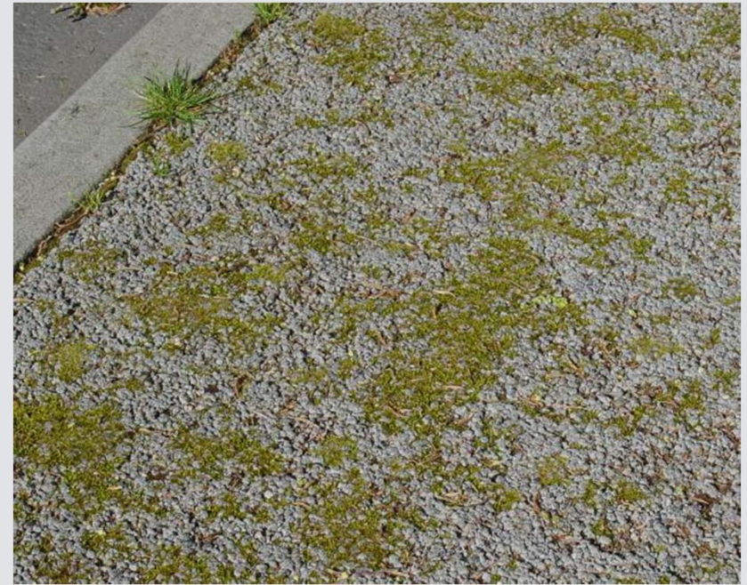
Above: Pervious Concrete City Sidewalk with moss
