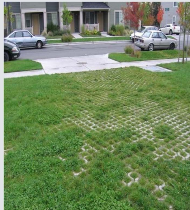
Maintenance road using TurfStone® over 1 ½" to 2" sand and 6" of crushed rock w/o fines
