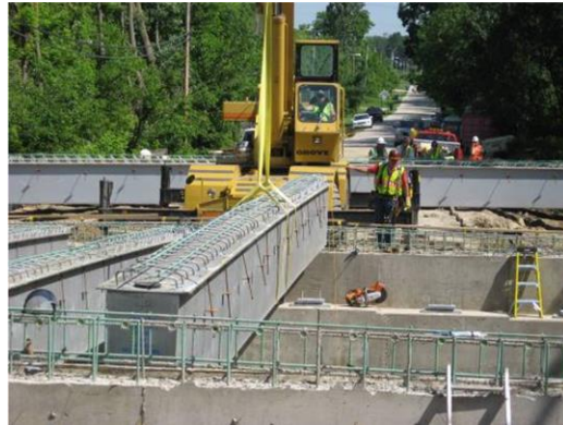
Figure 4. Erecting HCB with 30 tonne Crane
