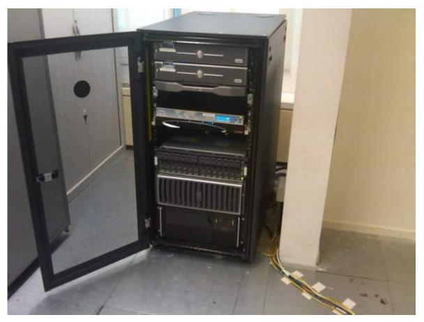
All non U.S. data centers replaced with this footprint. Acts as cloud capacity to move applications and services around the planet. Lots of empty rooms..... Fully remotely managed. What we call a DRiB.
