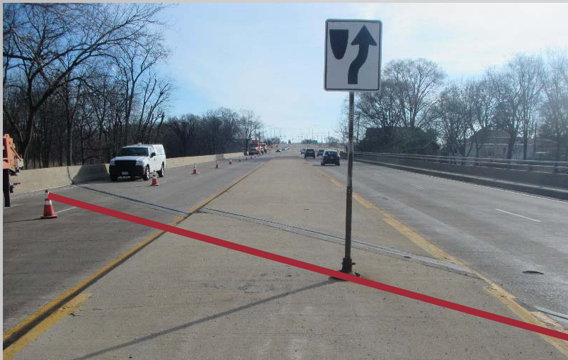
Successful retrofit of extreme skew joint in Illinois
