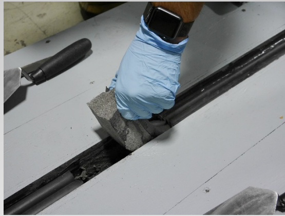
Remove damaged material
