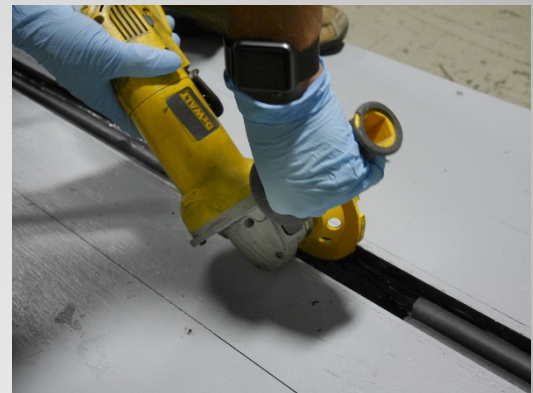
Grind substrate to remove remaining materials
