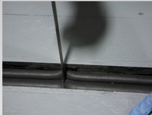
Cut on either side of damaged area
