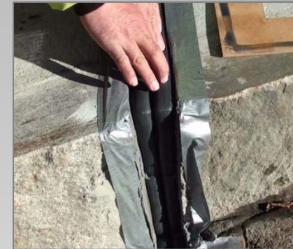
Inserting factory fabricated transitions
