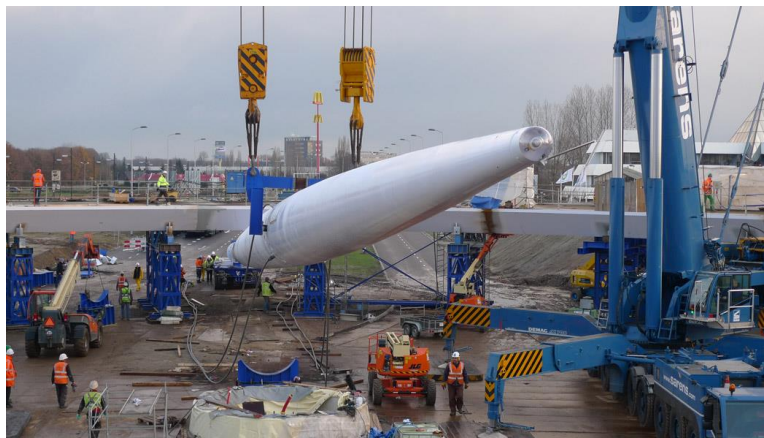
Fig. 9 Construction work on erecting the pylon
