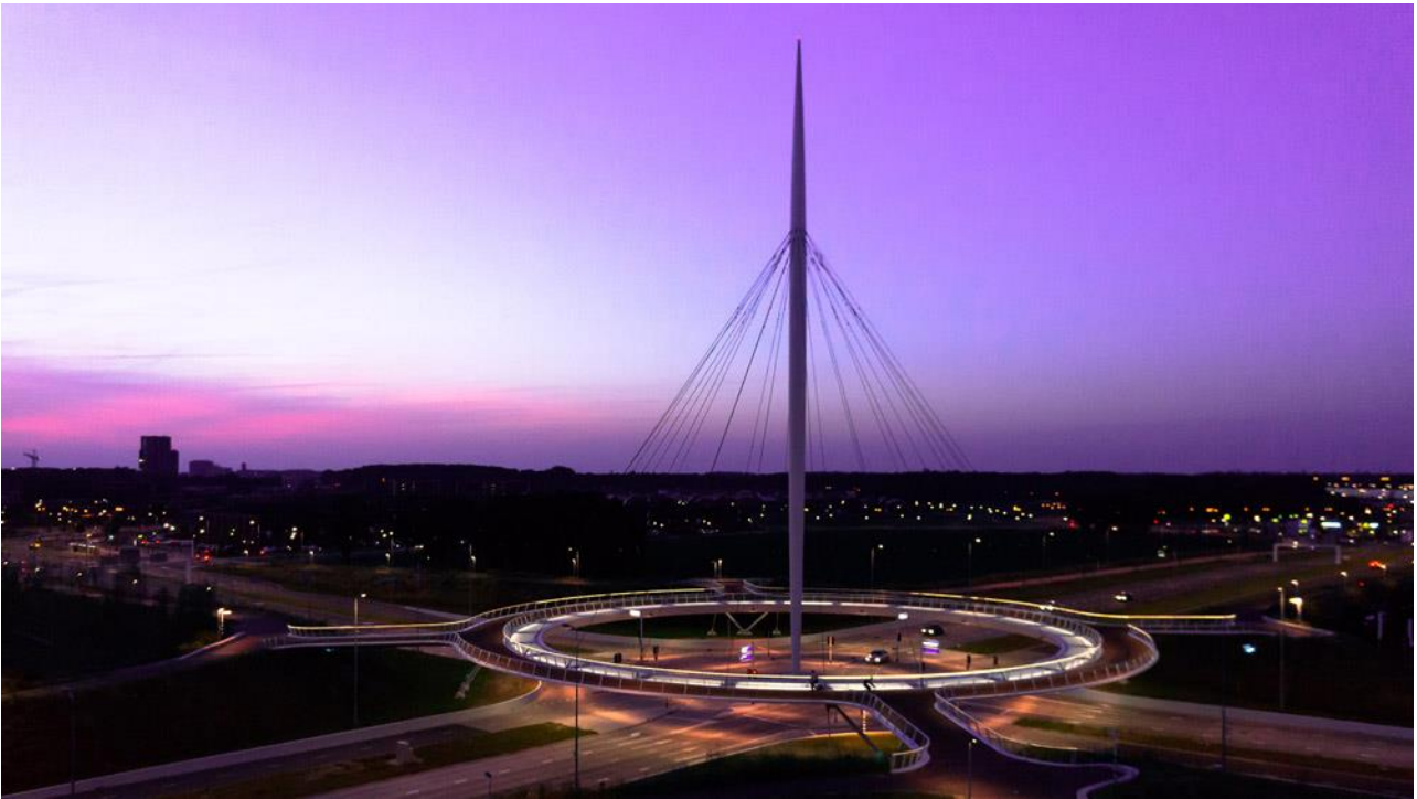
Fig.1 Aerial overview of the Hovenring by night
