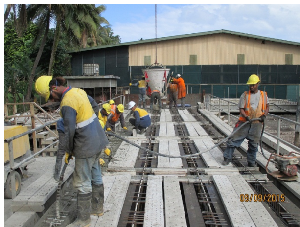
Figure 6. Precasting operations in the Suva yard.
