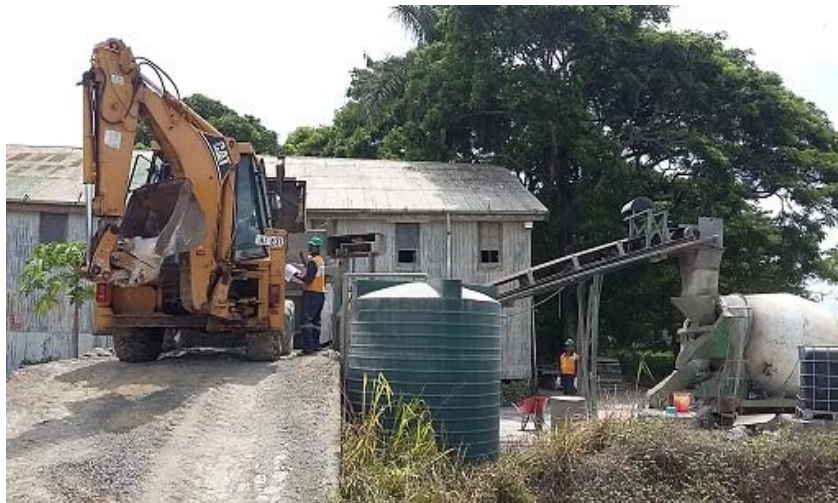
Figure 8. Concrete batching plant in Labasa.
