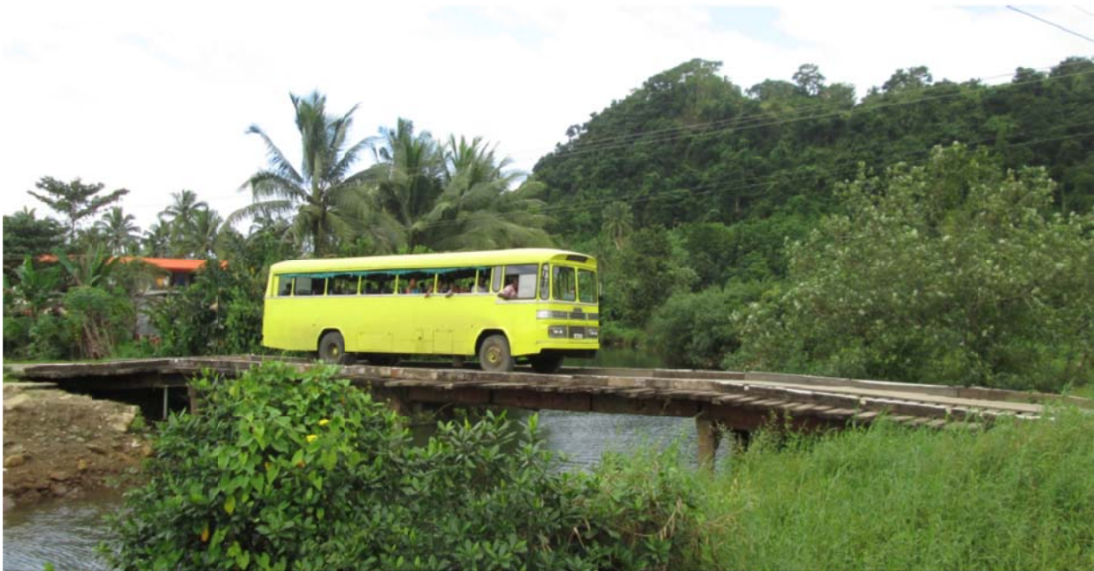
Figure 2. Existing Vunidilo bridge.
