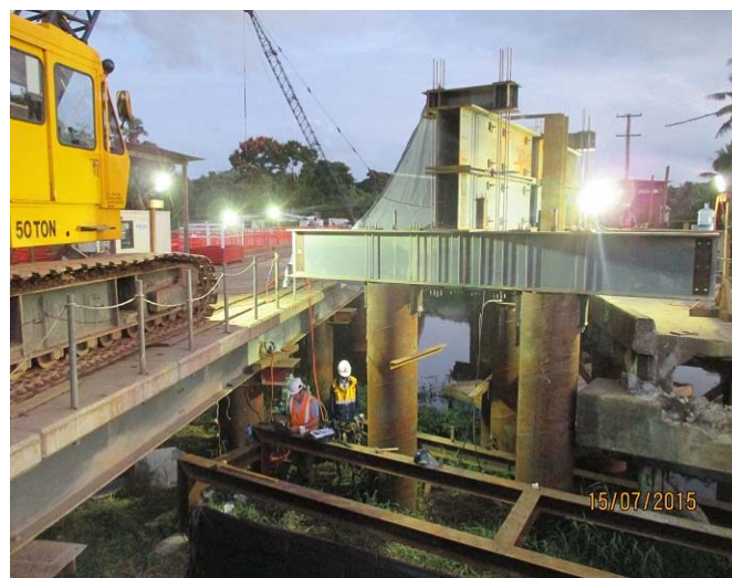
Figure 7. Pile load testing at Vunivaivai.
