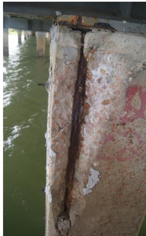
section losses were noted in the headstock stiffeners, these are elements that are only critical for jacking up the bridge during bearing replacement activities – something that is not likely to occur now the majority of the bearings have been fixed retrospectively.
