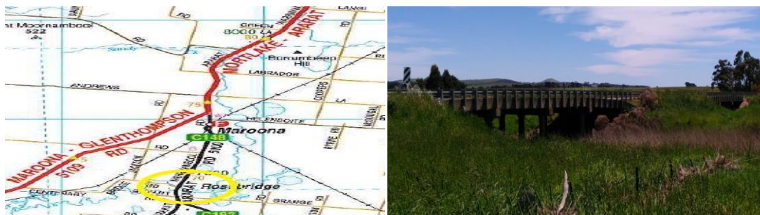
Figure 1. Location of Works and picture of site
