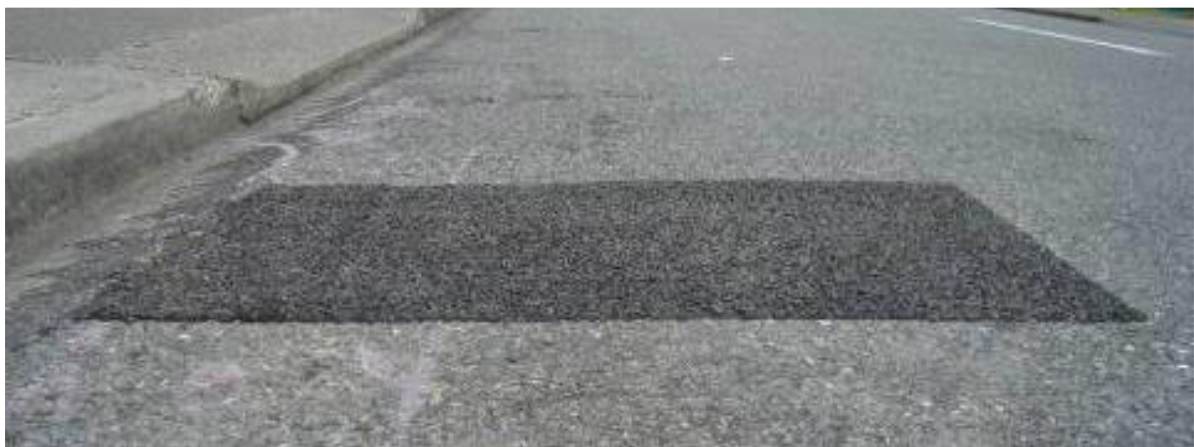
Image 4 : BRP Road Patch
