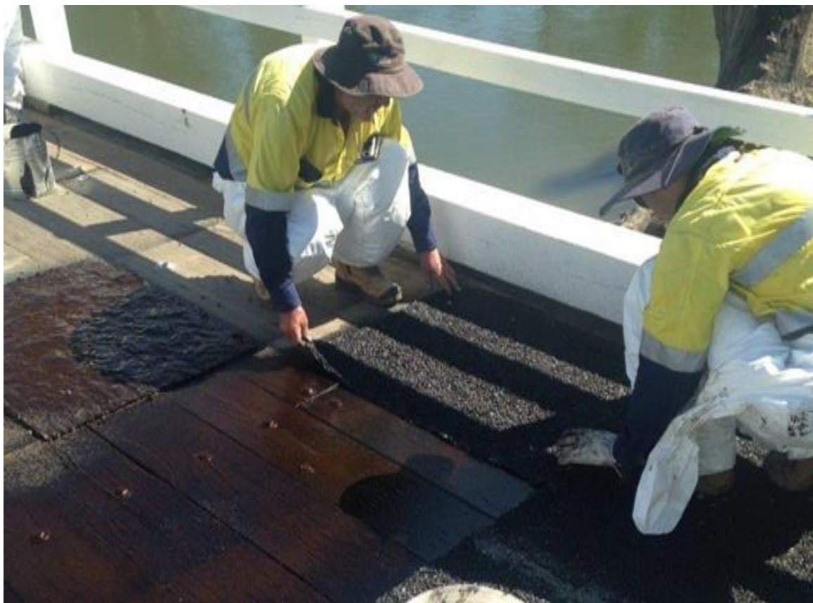
Image 7: Boundary Rod Bridge Pre Upgrade works June 2015 & BRP Installation
