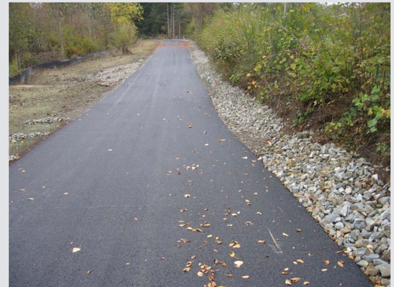
Porous Asphalt Drive, Pierce County
