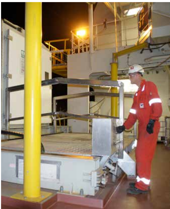
A hydraulic slide moves the evacuation system into cantilevered position for deployment.
