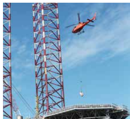
Removal of existing structure by helicopter
