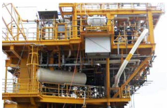
The container protects the evacuation chute against all types of weather
