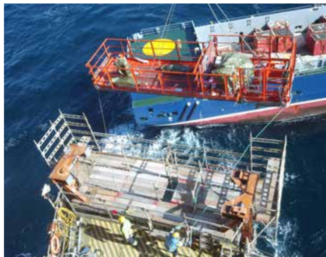
Davit sections - fully function tested onshore - replaced offshore
