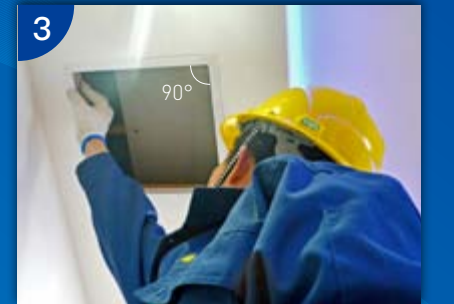
INSTALLING FRAME
