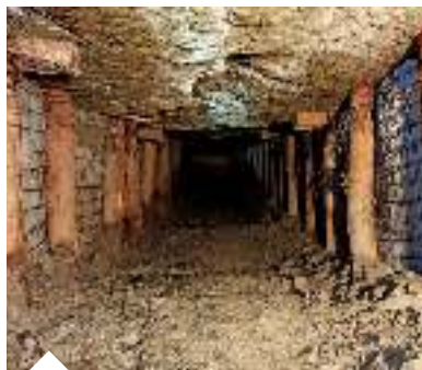
Stope supported with Conbex backfill
