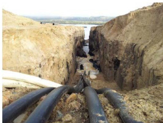
Figure 10. PE100 pipes used to dewater the mine
