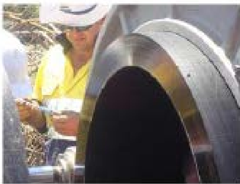
Figure 8. Butt Welding of 1,000 mm diameter pipes in the field
