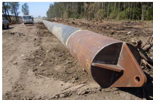
Figure 9. A 300 meter long length of pipe prepared for HDD installation
