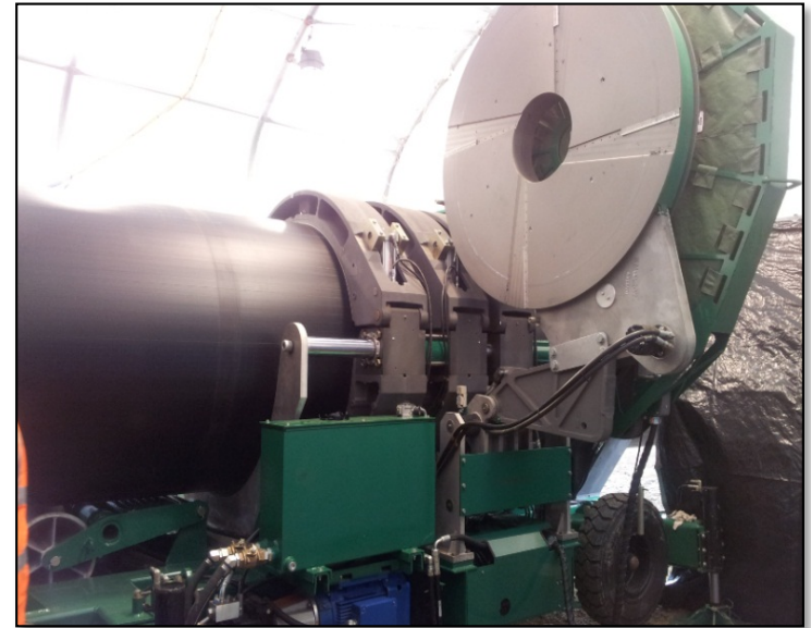
Butt Welding in the Field
