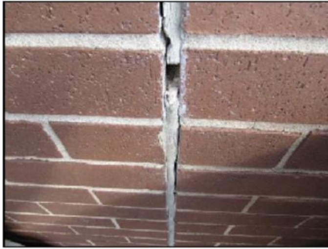
P10 - Brick Control Joint
