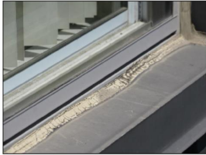
P5 - Single Glazed Window and Metal Sill Flashing
