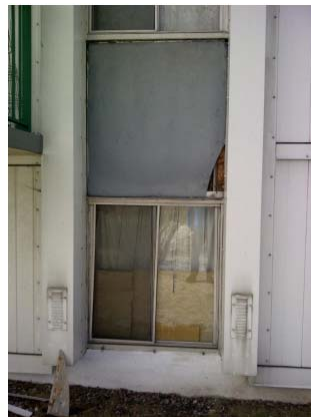
Photo 4: Trial transit panel removal at ground floor unit - transit panel could not be removed without removing adjacent metal cladding or breaking the panel.
