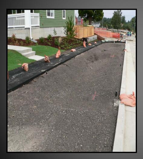
Construction activity sloping to bioretention facility
