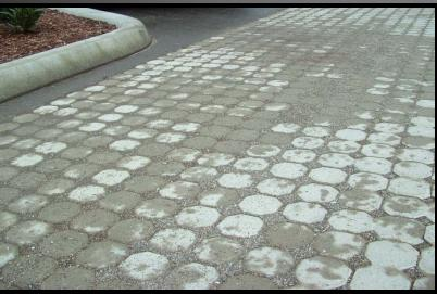
Roads (permeable pavers are used for construction access)
