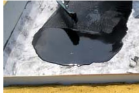
American Hydrotech MM6125 monolithic fluid applied rubberized asphalt membrane
