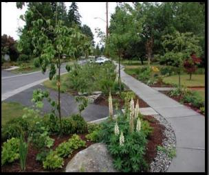
Integrated engineered, small scale stormwater controls.
