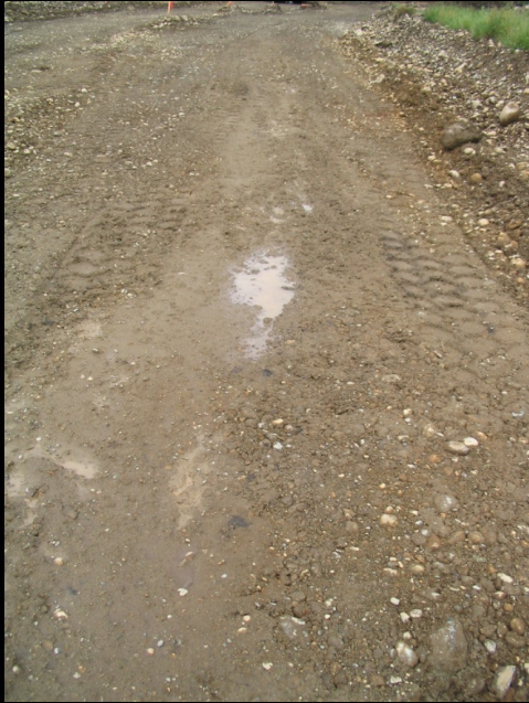
Compacted subgrade
