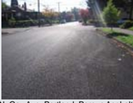
N. Gay Ave, Portland. Porous Asphalt Concrete (2005 - 8" porous AC over 6" Subbase)
