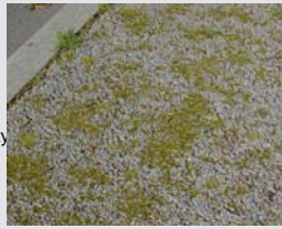
Above: Pervious Concrete City Sidewalk with moss
