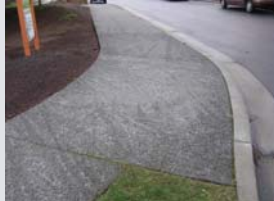
Staining from compost spilling onto pervious concrete.
