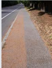
Photos from Maintenance Memo from Craig Tosomeen, City of Olympia Photos from Maintenance Memo from Craig Tosomeen, City of Olympia using Leaf/Litter Vacuum (Minuteman Parker Vac-35) September 2006 to clean pervious concrete sidewalk installed in 1999.
