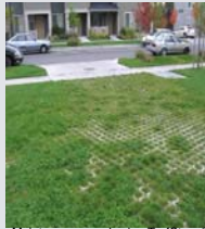
Maintenance road using TurfStone ® over 1 1/2" to 2" sand and 6" of crushed rock w/o fines
