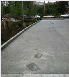
Patching due to footprint indentation.
