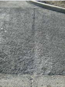
Pavement was placed early and used as a construction entrance for concrete deliveries.
