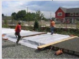
Pavement being covered immediately as it's being placed to hold moisture in for curing.
