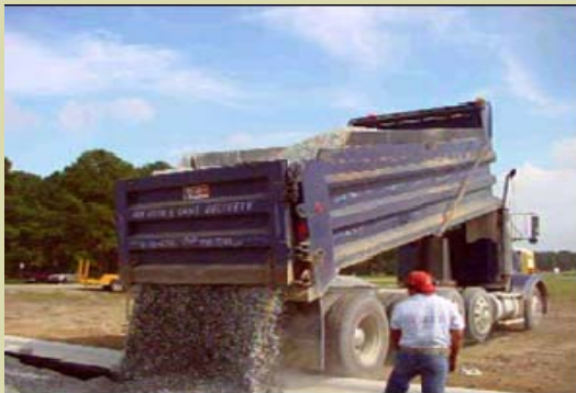
Keep delivery trucks off of native soil, if at all possible
