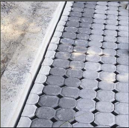
Edge pavers cut and placed, then compacted
