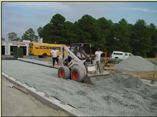
Final grading of base material
