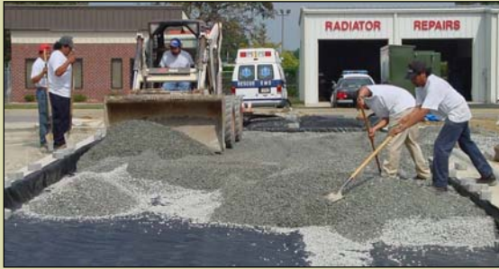
Spreading Base Material – “back-dumping”
