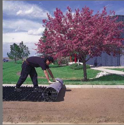
2. Unroll paver, connect and cut as needed
