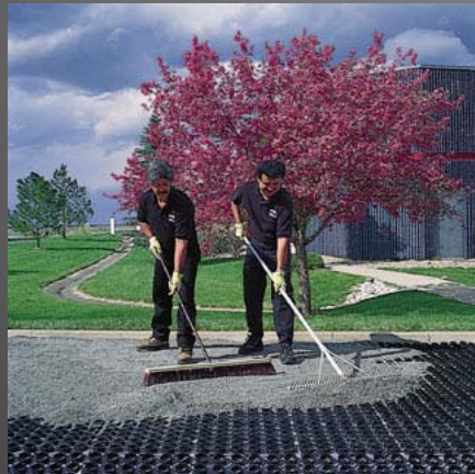
4. Fill with open graded 3/8" aggregate (gravel)
