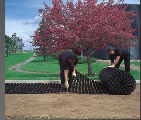
3. Unroll paver, connect, and cut as needed
