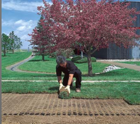
5. Lay sod or hydroseed
