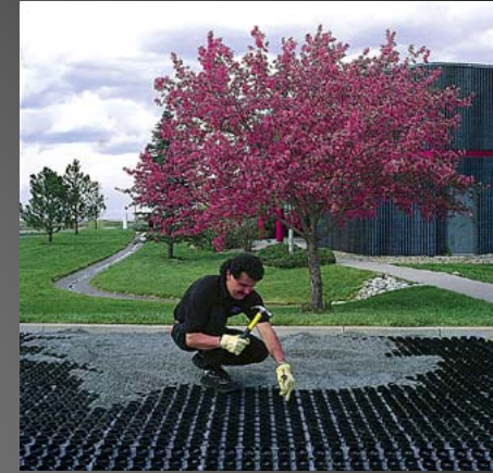
3. Secure to base with anchors*
